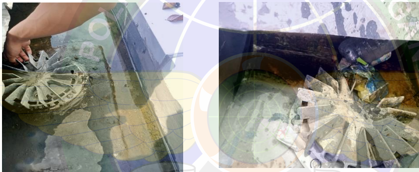
Gambar 4. 16 Roof Drain Terminal
