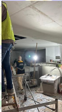
Gambar 23 Monitoring proyek tenant Terminal 2
