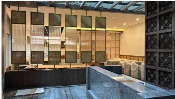
Gambar 32 Monitoring proyek tenant blue sky Terminal 2
