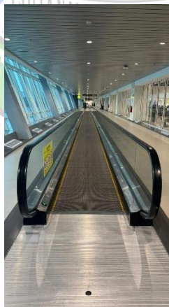
Gambar 11 Monitoring Travalator area koridor Terminal 1
