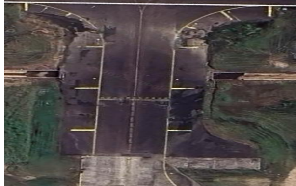
Gambar 4 7 (Taxiway Charlie Bandara Juwata)
