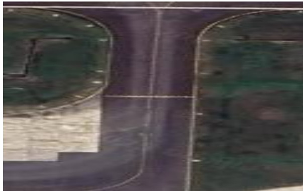
Gambar 4 5 ( Taxiway Alpha Bandara Juwata )
