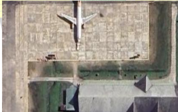
Gambar 4 3 (Main Apron East Bandara Juwata)
