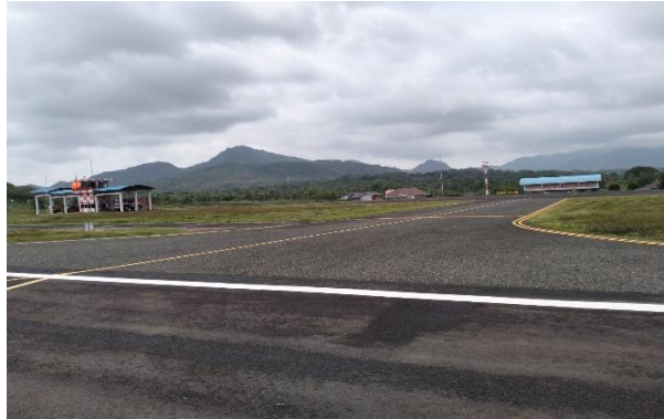
Gambar 4. 3 Taxiway Bandar Udara Harun Thohir
