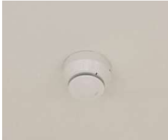
Gambar 3. 7 Smoke detector
