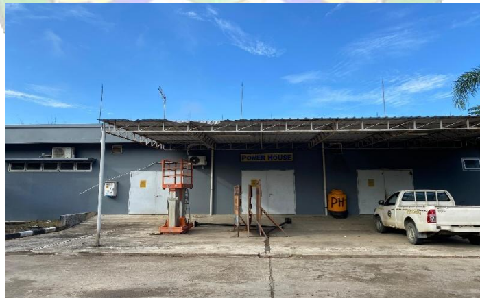
Gambar 4. 8 Gedung Power House
