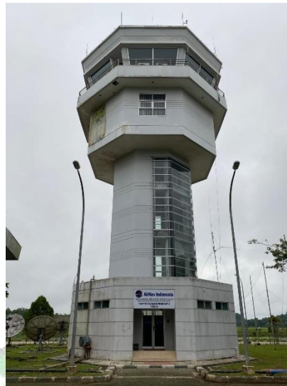
Gambar 4. 7 Menara Air Traffic Controller (ATC)
