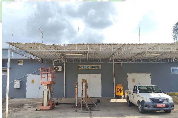
Gambar 4. 12 Gedung Power House
