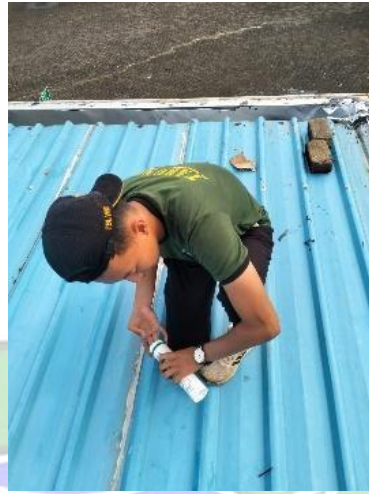
Gambar 4. 15 Pemberian Silicone Sealant
