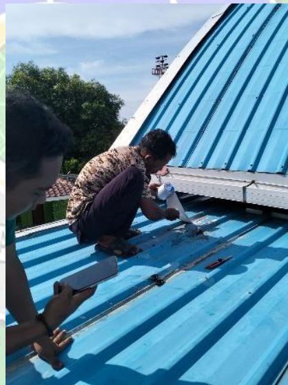
Gambar 4. 16 Proses Penambalan Atap Terminal
