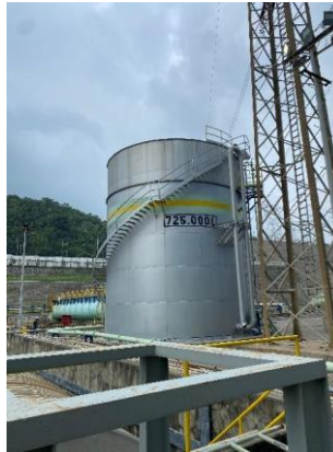
Gambar 3. 16 Demin Water Tank
