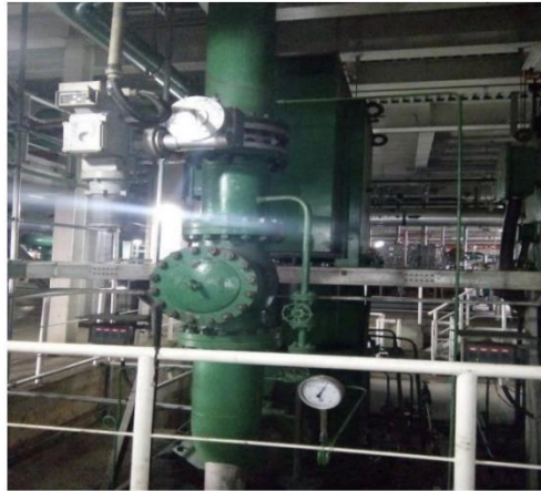
Gambar 3. 18 Condensate Pump
