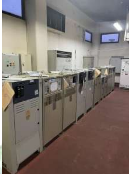
Gambar 3. 2 Constant Current Regulator (CCR)
