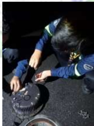
Gambar 4. 4 Proses Membuka Cover Lampu Runway Edge Inset
