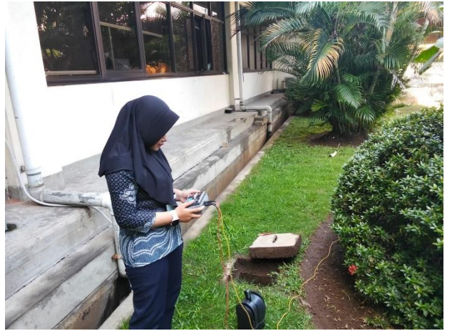
Grounding Gedung AirNav
