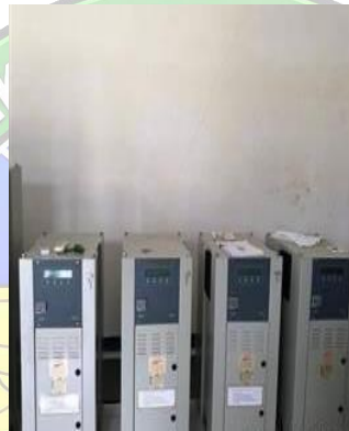
Gambar 3.1.5 12 Constant Current Regulator
