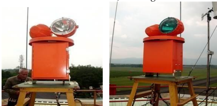
Gambar 3.1.5 10 Rotating Beacon
