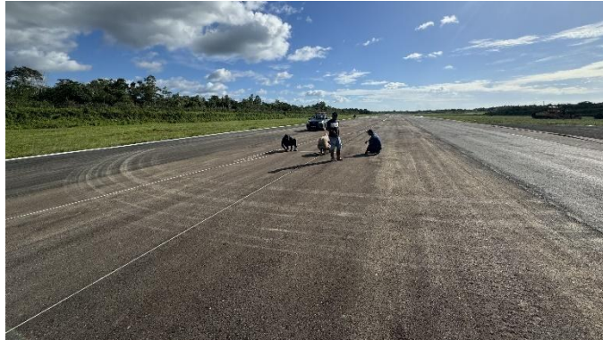
Gambar 4.58 Pengukuran Dimensi Marka Runway Designator
