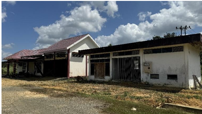
Gambar 4.21 Gedung Power House
