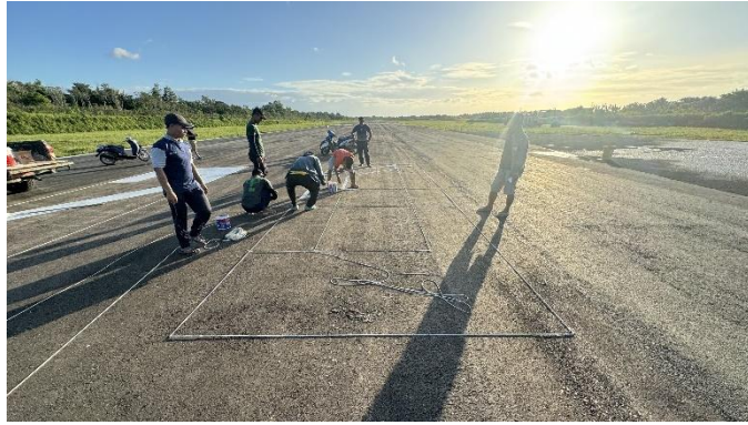
Gambar 4.63 Pengecatan Marka Runway Designator
