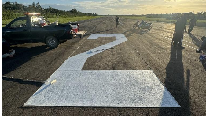
Gambar 4.65 Marka Runway Designator
