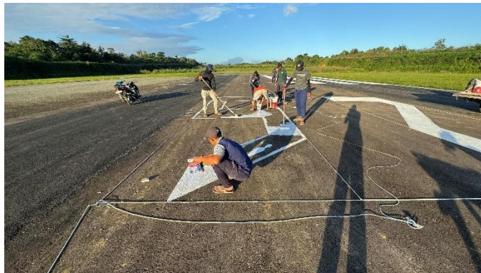
Gambar 4.64 Pengecatan Marka Runway Designator
