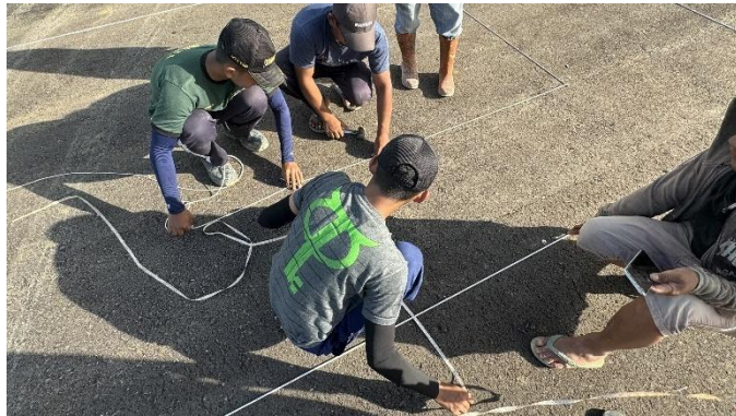
Gambar 4.59 Pengukuran Dimensi Marka Runway Designator
