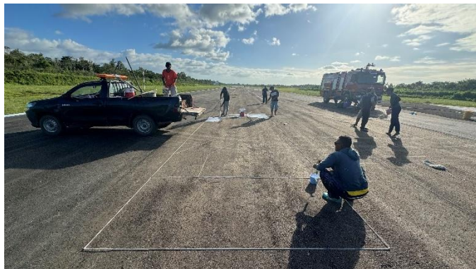
Gambar 4.62 Pengecatan Marka Runway Designator
