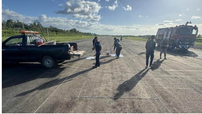
Gambar 4.61 Pengecatan Marka Runway Designator
