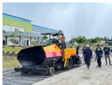
Gambar 4.17 Asphalt Finisher
