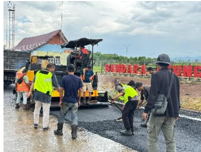
Gambar 4.28 Trial Compaction
