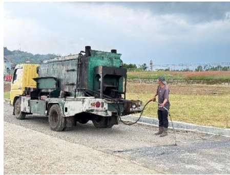
Gambar 4.16 Mobil Asphalt Sprayer
