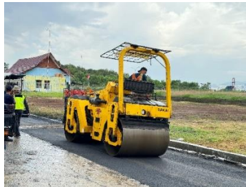
Gambar 4.19 Tandem Roller
