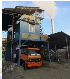
Gambar 4.17 Asphalt Mixing Plant (Sumber : Dokumentasi Penulis)
