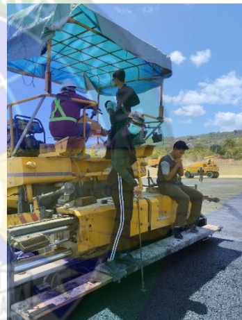
Penghamparan Aspal AC-BC di area perpanjangan runway
