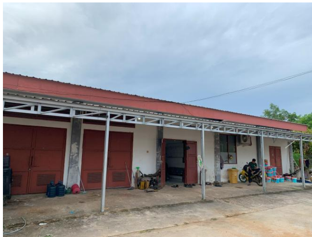
Gambar 4. 10 Power House (PH)
