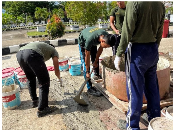
Gambar 4. 43 Perataan Campuran Beton
