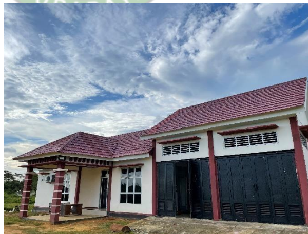
Gambar 4. 6 Gedung Power House
