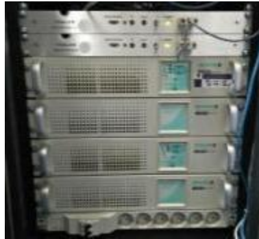
Gambar 3.45 Receiver ADS-B
