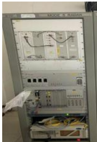
Gambar 3.42 Transmitter Radar MSSR
