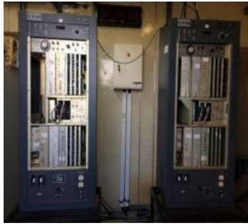
Gambar 3.40 Transmitter T-DME
