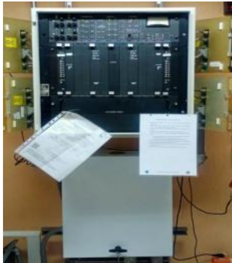
Gambar 3.29 Transmitter Localizer
