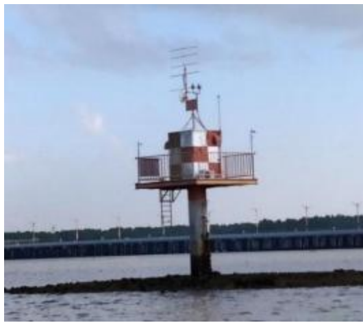
Gambar 3.38 Ground Station Middle Marker
