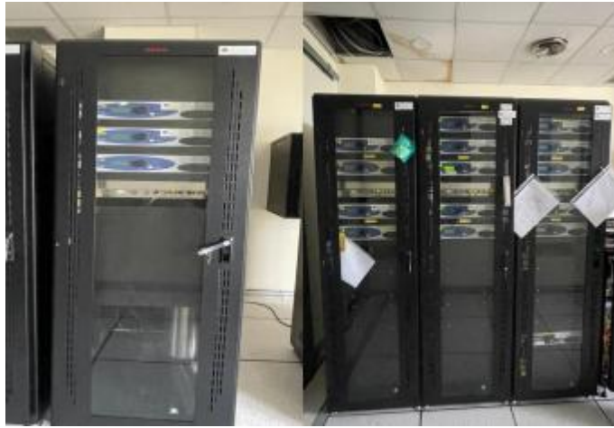
Gambar 3.12 Radio VHF Receiver
