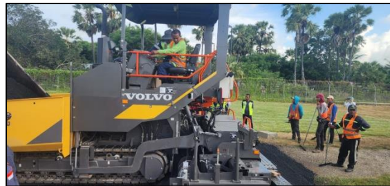
Gambar 4. 27 Asphalt Finish
