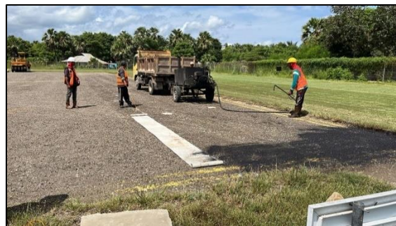
Gambar 4. 28 Asphalt Sprayer
