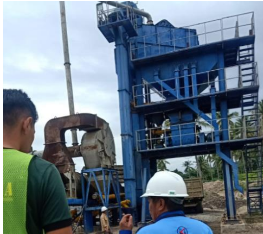
Gambar 4. 26 Asphalt Mixing Plant (AMP) (Sumber : Dokumentasi Pribadi, 2024)
