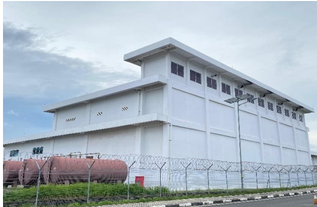
Gambar 4.3 Gedung Power House
