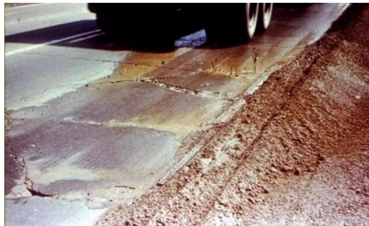
Gambar 3. 4 Merembesnya Air (Sumber: Slideshare.Net/Aguskerusakan-Perkerasan-Kaku )
