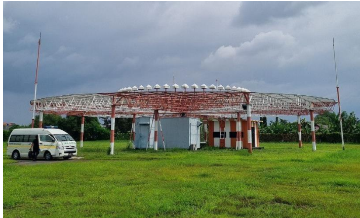
Gambar 3.3. 1 Ground Station DVOR
