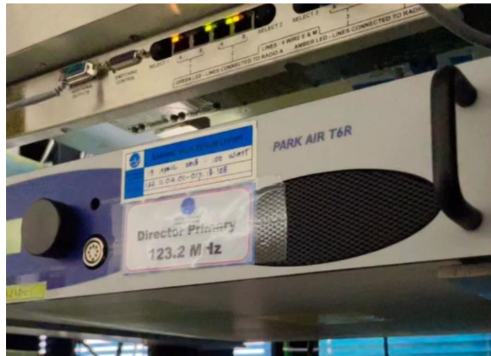
Gambar 3.10. 1 Frequency director 123,2 Mhz terjadi interference ATIS
