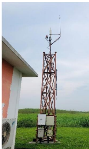
Gambar 3. 21 Antenna Peralatan RU (Remote Unit) MLAT
