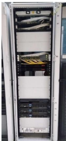
Gambar 3. 22 Rak Server ASMGCS di Equipment Room
