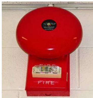
Gambar 3. 10 Fire Alarm Bell
