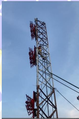
Gambar 3 .16 Antena Glide Path
