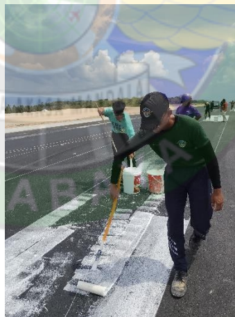
Gambar 4. 24 Pengecatan Marka Threshold
