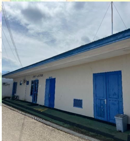
Gambar 4. 7 Gedung Power House
