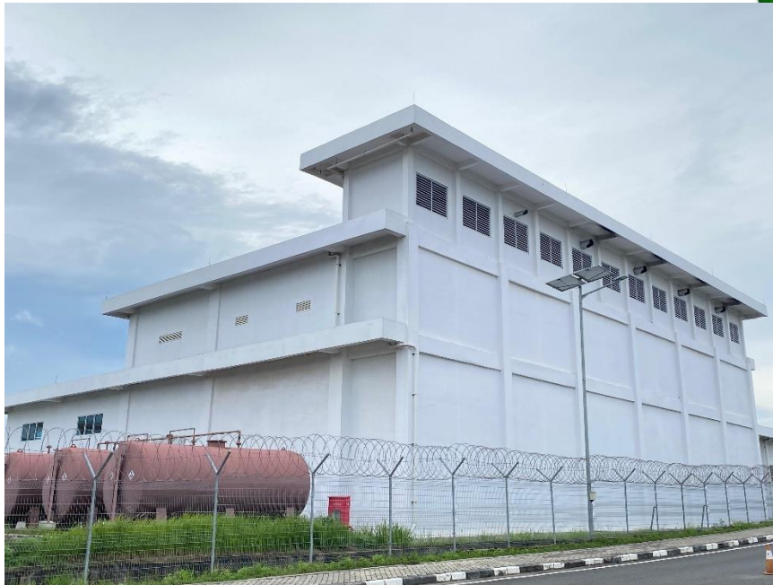
Gambar 4. 5 Gedung Power House (PH)
