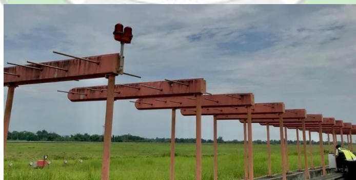
Gambar 3 . 11 Antenna Localizer 03
