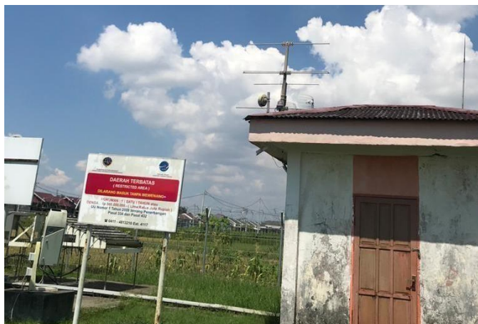
Gambar 3 . 27 Shelter Marker Beacon 13
