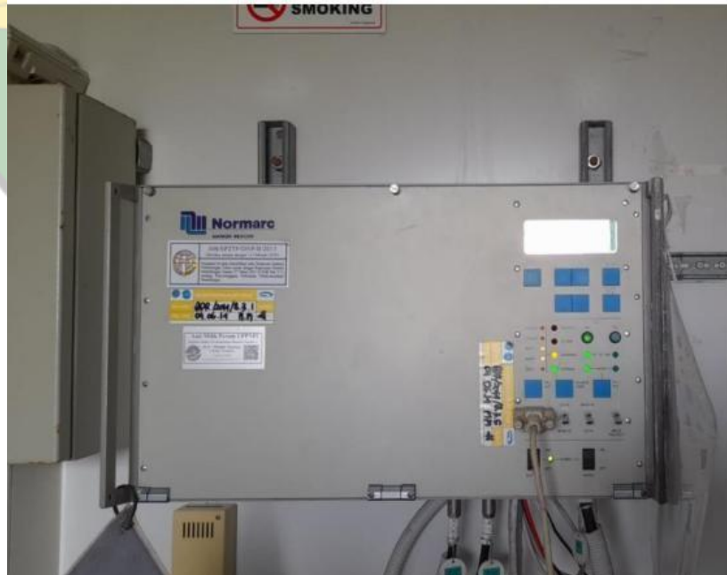
Gambar 3. 10 Peralatan Middle Marker Merk NORMAC
