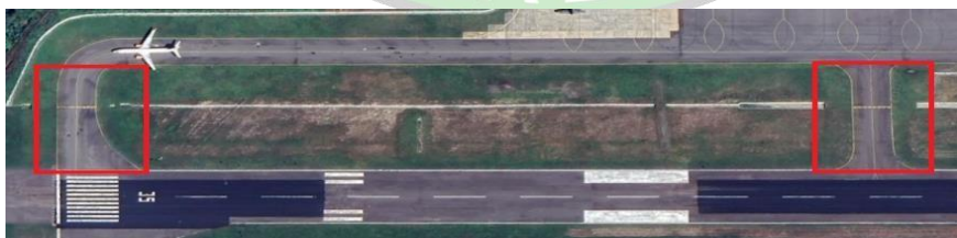
Gambar 3. 2 Taxiway Komodo Airport
