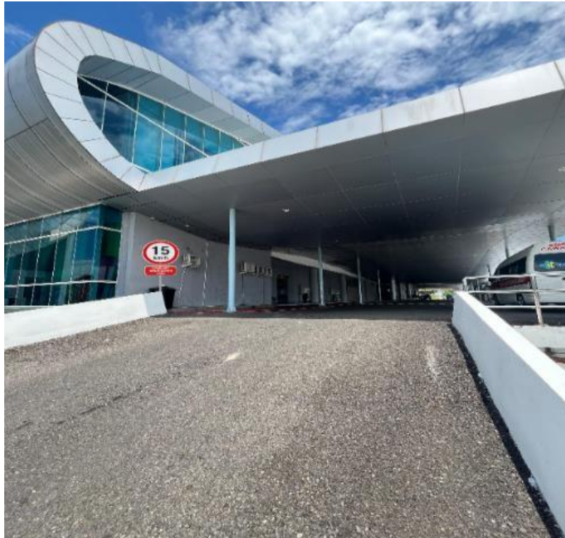
Gambar 4. 12 Implementasi Sign Maksimum Speed di Area Make-Up / Break down Area
