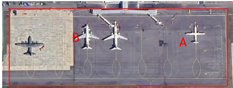
Gambar 3.3 Apron Komodo Airport
