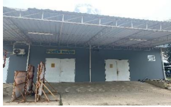
Gambar 2.6 Gedung Power House
