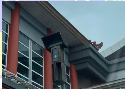
Gambar 2. 36 Advance Docking Guidance System (ADGS)
