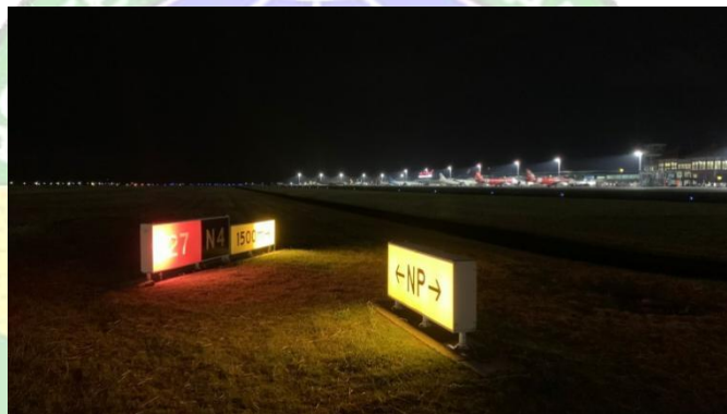
Gambar 2. 34 Movement Area Guidance Sign (MAGS) Sumber : Dokumentasi Penulis
