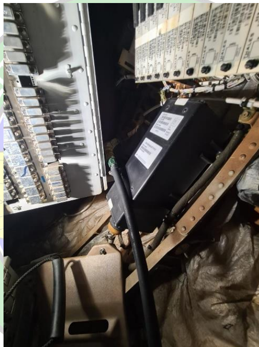
Gambar 4. 16 Flushing Static Pressure Lines
