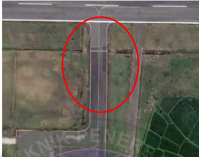
Gambar 4.10 Landasan Hubung ( Taxiway )
