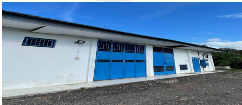
Gambar 4.4 Gedung Power House
