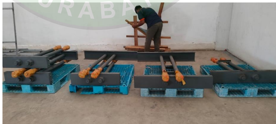
Gambar 4. 32 Bolt Anchor
