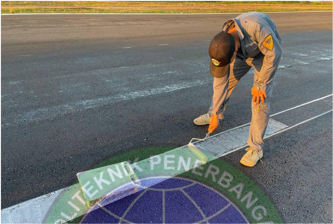
LAMPIRAN 17 : Pngecatan Marka Runway ( Centerline )
