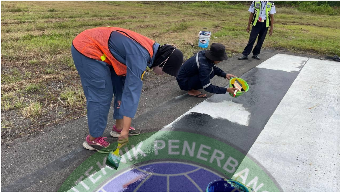
LAMPIRAN 3 : Pengecatan Marka ( Threshold )
