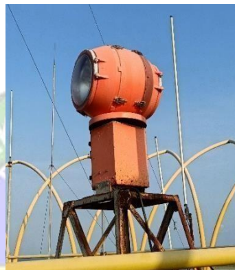
Gambar 2 19 Rotating Beacon
