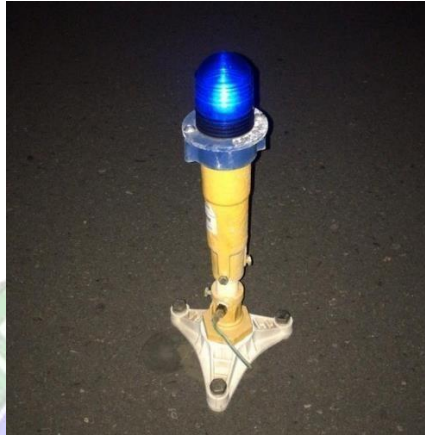
Gambar 2 10 Taxiway Edge Light
