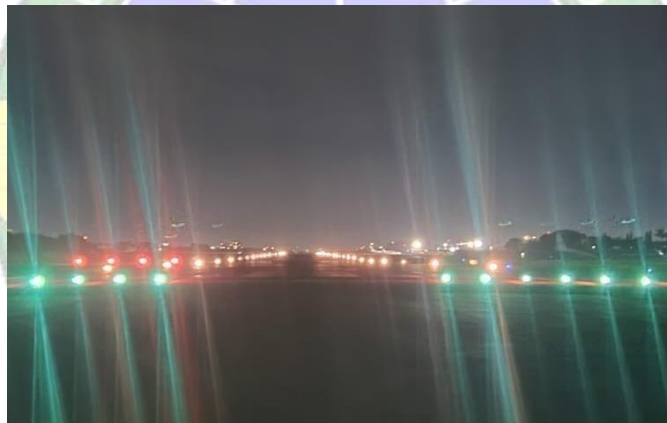
Gambar 3 1 Airfield Lighting System
