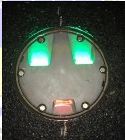
Gambar 2 6 Threshold dan Runway End Light
