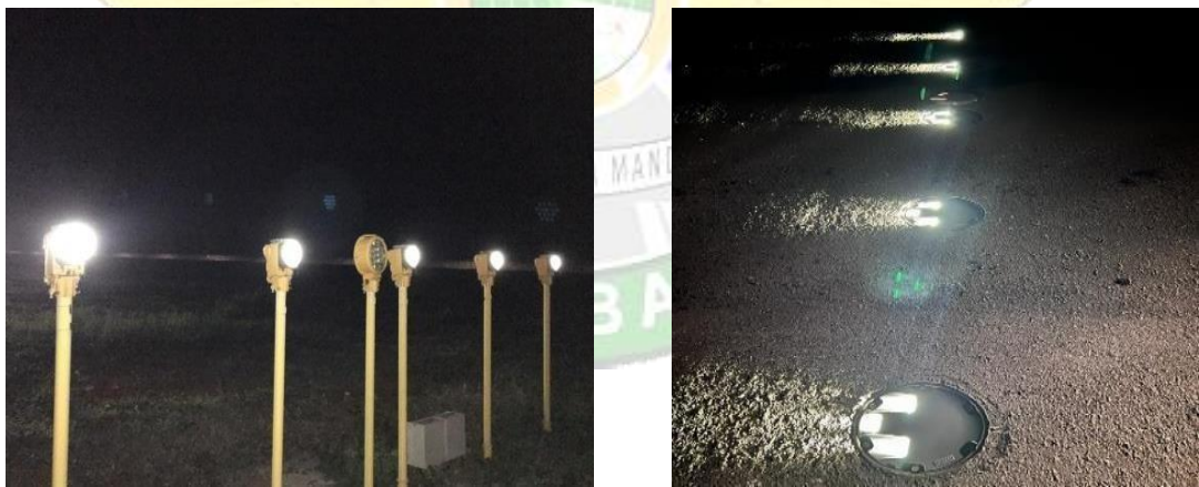
Gambar 2 2 Approach Lighting System
