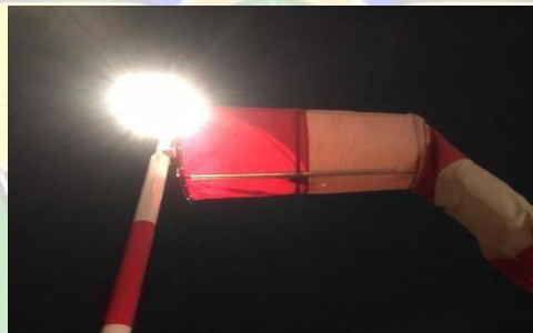
Gambar 2 14 Wind Direction Indicator (WDI)
