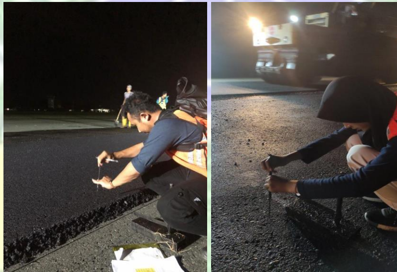
Lampiran 2 Pengukuran Ketebalan Asphalt
