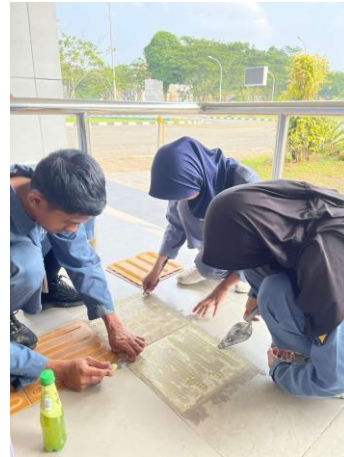
Perbaikan guilding block disabilitas
