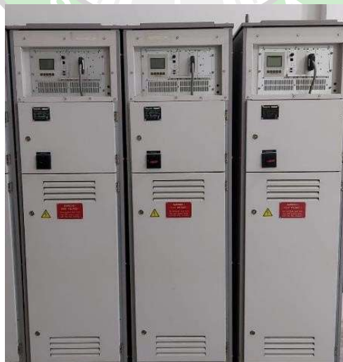
Gambar 2. 22 CCR (Constant Current Regulator)
