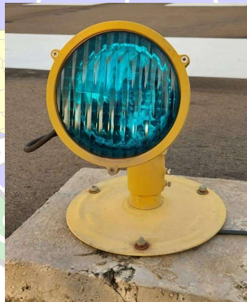
Gambar 2. 19 Runway Threshold Light
