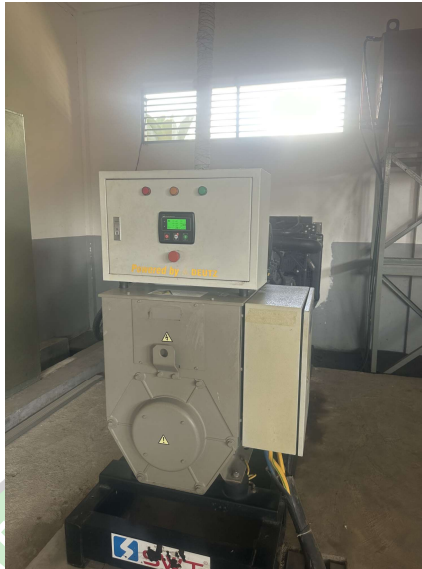
Gambar 3. 8 Alternator
