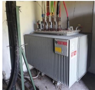
Gambar 2. 35 Transformator
