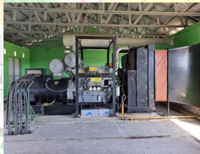
Gambar 2. 34 Generator Set 750 kVA
