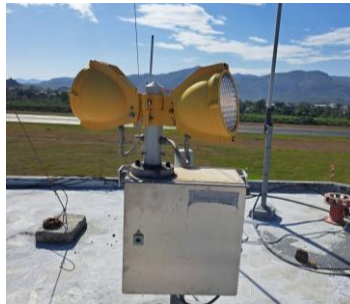
Gambar 2. 23 Rotating Beacon
