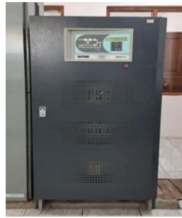
Gambar 2. 37 Uninterruptible Power Supply (UPS)
