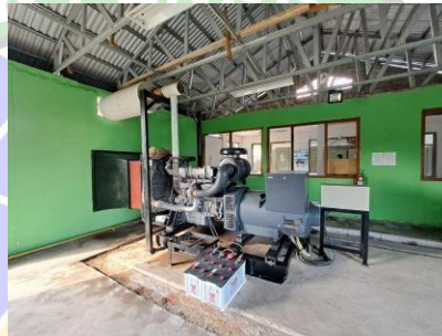
Gambar 2. 32 Generator Set 250 kVA
