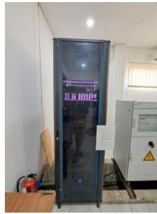
Gambar 2. 28 Marshalling Cabinet
