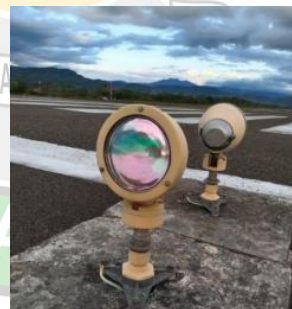
Gambar 2. 21 Threshold Light
