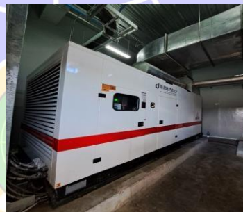
Gambar 2. 33 Generator Set 500 kVA
