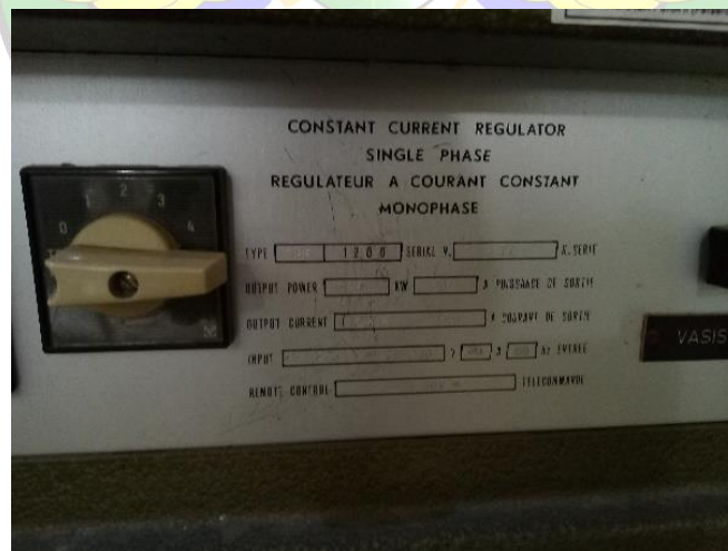
Gambar 2. 34 CCR Precision Approach Path Indicator (PAPI) II
