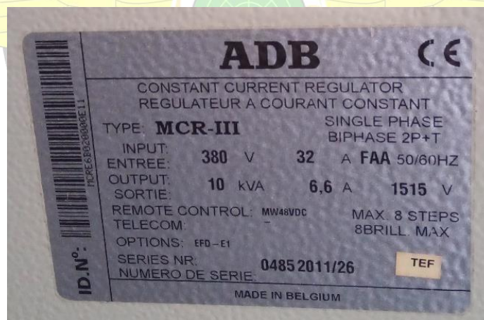
Gambar 2. 30 CCR Medium Approach Light System (MALS)
