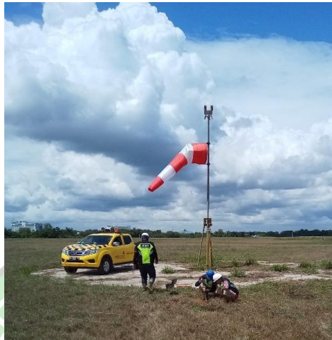
Gambar 2. 26 Wind Direction Indicator
