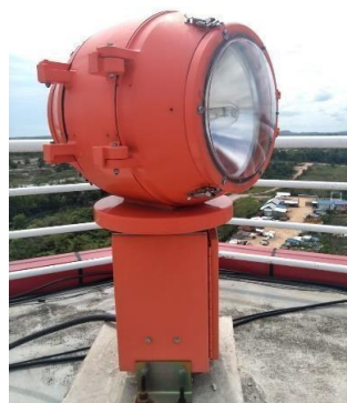
Gambar 2. 27 Rotating Beacon
