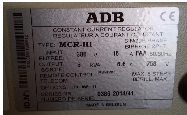
Gambar 2. 37 CCR Taxiway Edge Light Rangkaian D
