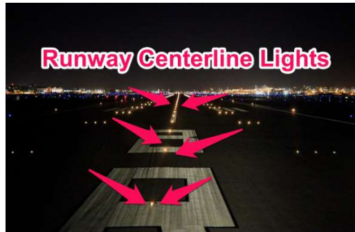
Gambar 3. 2 RCL (Runway Centerline Light) Sumber : Google Image
