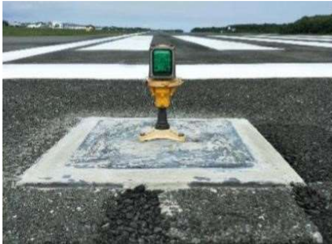
Gambar 4. 11 Threshold Light Elevated Sumber : Hasil Karya Penulis
