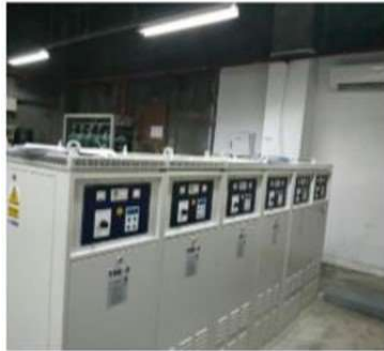
Gambar 3. 4 Constant Current Regulator
