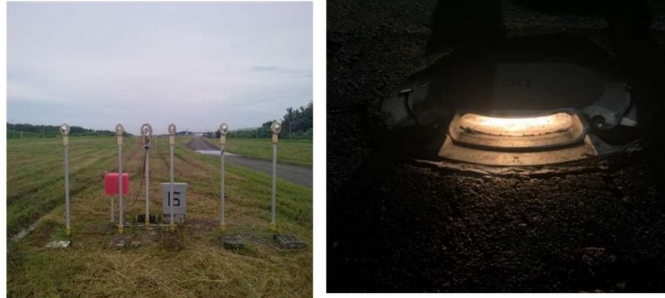
Gambar 4. 5 Approach Light Elevated & Inset Sumber : Hasil Karya Penulis
