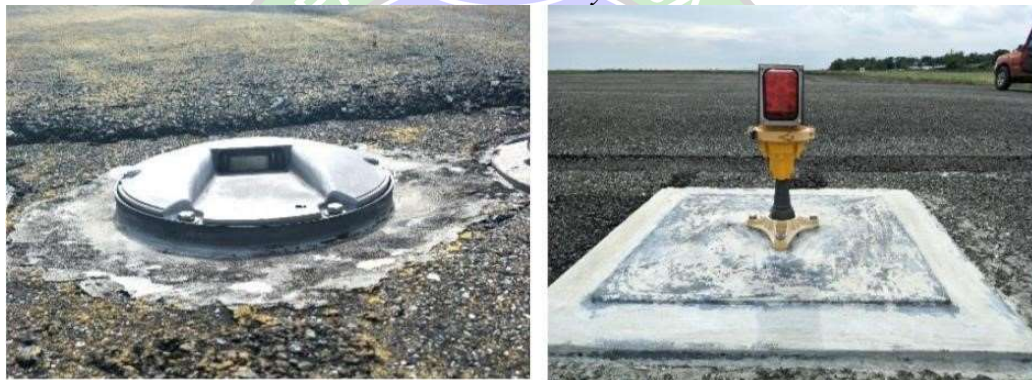
Gambar 4. 12 Threshold Light Inset & Runway End Light Sumber : Hasil Karya Penulis
