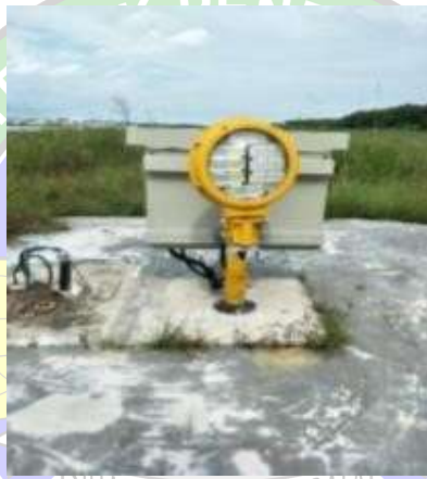
Gambar 4. 7 Runway Threshold Identification Light (RTIL) Sumber : Hasil Karya Penulis
