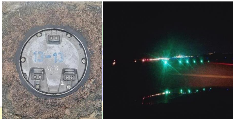
Gambar 2. 15 Threshold light
