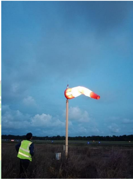
Gambar 2. 24 Wind Direction Indicator (WDI)
