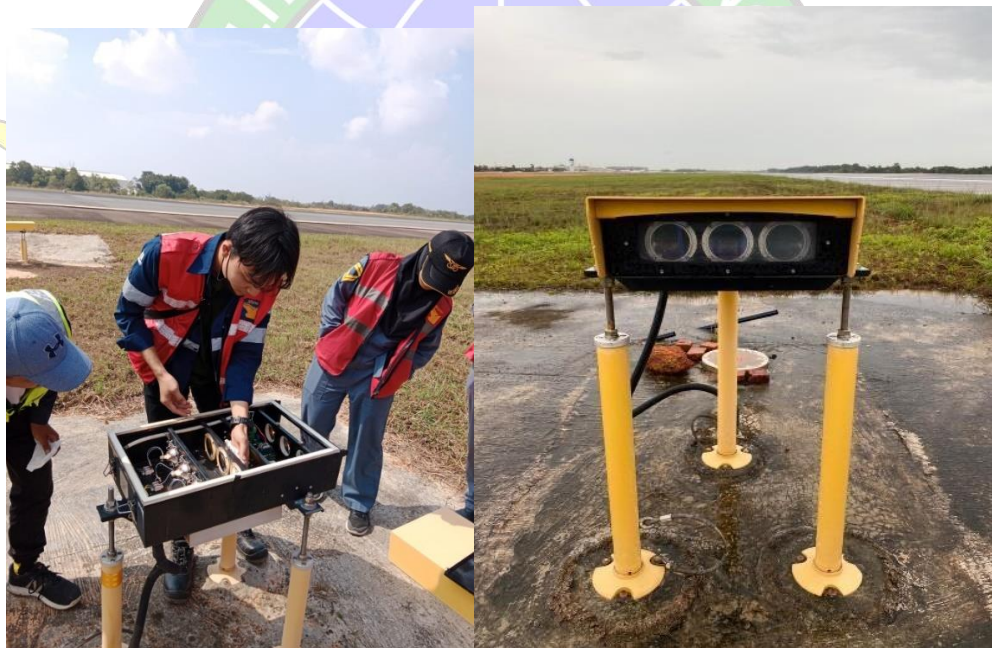
Gambar 2. 10 Precision Approach Path Indicator (PAPI)
