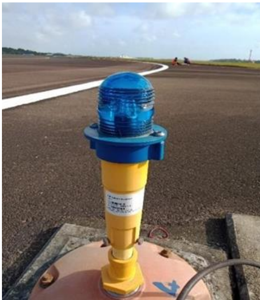
Gambar 2. 12 Turning Area Light
