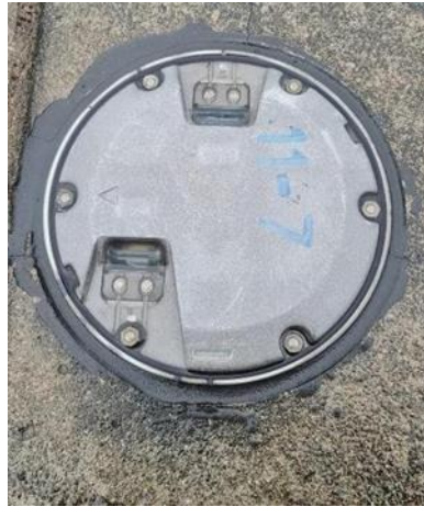
Gambar 2. 14 Runway Edge Light insert
