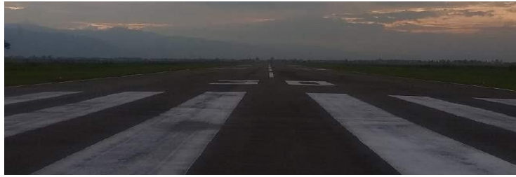
Gambar 4. 1 Runway Bandara Depati Parbo
