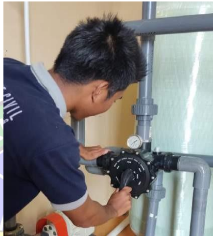
Gambar 4. 41 Proses Backwash System
