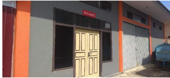
Gambar 4. 12 Gedung Power House
