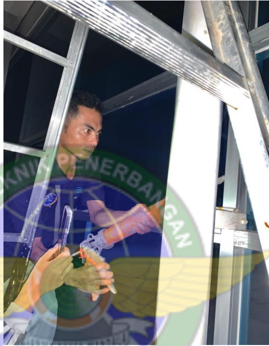
Gambar 4. 43 Proses Pemberian Silicon Sealant
