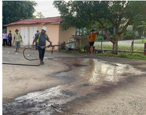
Gambar 4. 28 Proses Penghamparan Tack Coat
