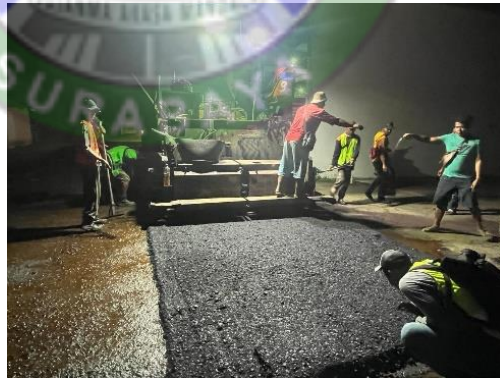
Gambar 4. 29 Proses Penghamparan Asphalt Hotmix
